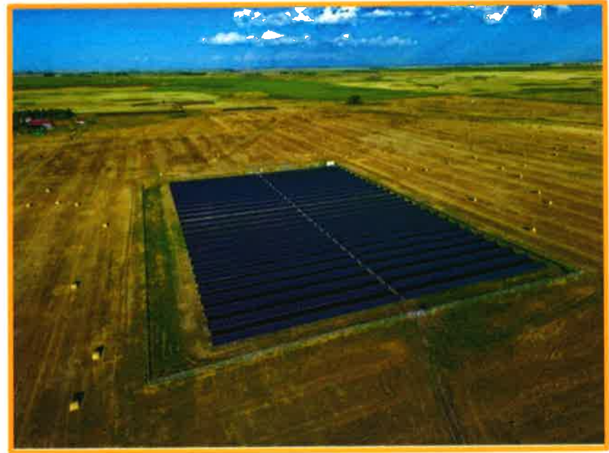
Example of a solar project – Compass Greenfield Development's NM Solar 2020 Inc., Lomond Saskatchewan – approximately 7 acres
